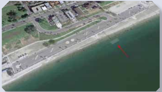
Aerial view of the Under Ocean Floor Seawater Intake and Discharge Project
