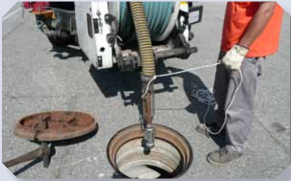
State-of-the-art video equipment utilized by Sewer Division staff
