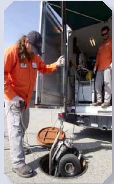
Robotic technology allows staff to pinpoint problems without expensive street excavations
