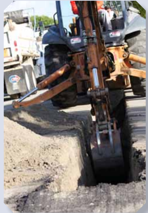
Crews work to replace old cast-iron mains throughout the city
