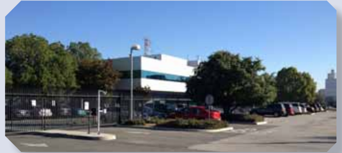
The new Emergency Operations Center (EOC) located next to the Groundwater Treatment Plant
